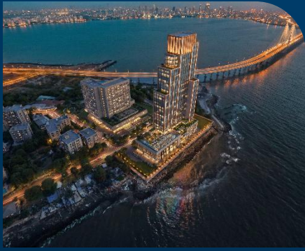
Taj Bandstand (Excavation completed) (2030)
