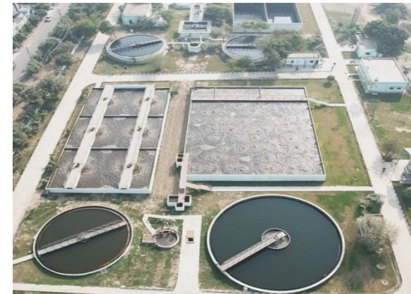
Upgradation of 5 MLD to 10 MLD CETP Rai Sonipat Haryana
