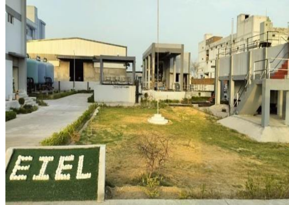
Upgradation of 16 to 26 MLD CETP Barhi Sonapat Harayana
