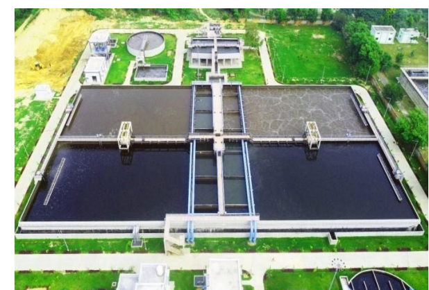
50 MLD Jalandhar Punjab
