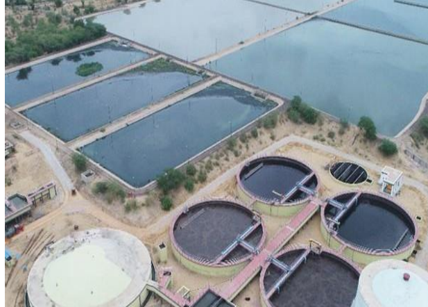
40+12 MLD STP Bikaner Rajasthan project ( includes Solar Plant)
