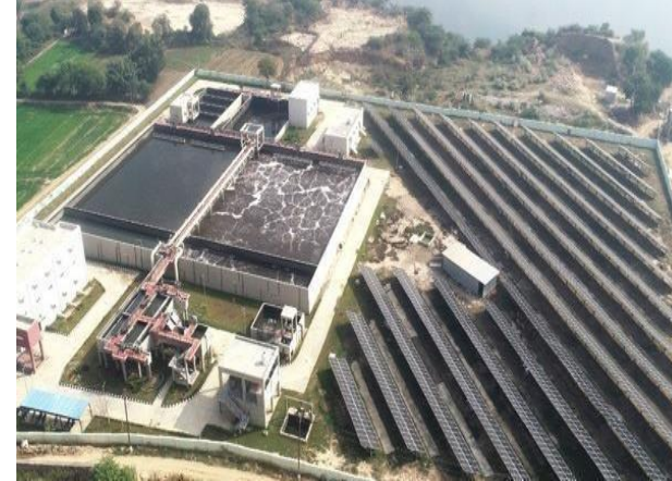
30 MLD STP Kota Rajasthan(Includes Solar Plant)
