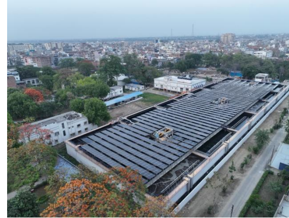
55 MLD STP, Varanasi, UP (includes solar plant)
