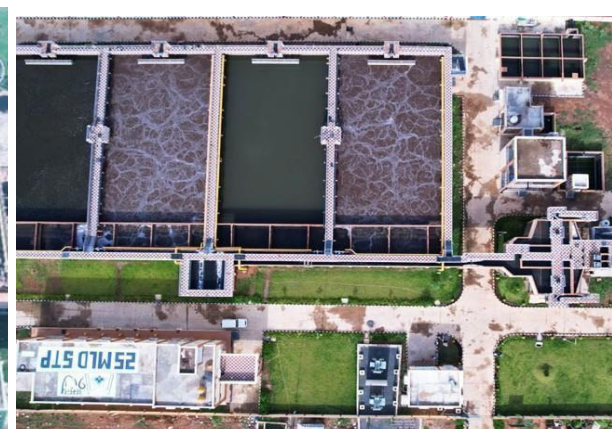
25 MLD STP, Jagdalpur, Chattisgarh
