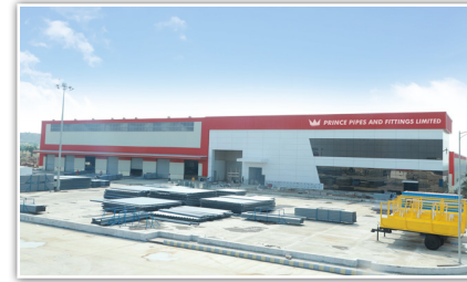
Jobner - Rajasthan (Pipes & Water Tanks)
