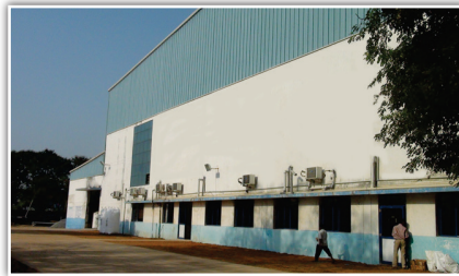
Chennai - Tamil Nadu (Pipes)
