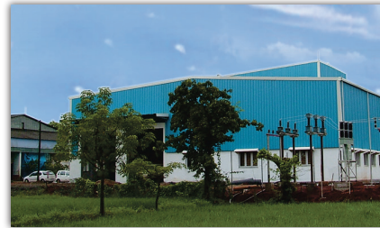
Kolhapur - Maharashtra (Pipes)
