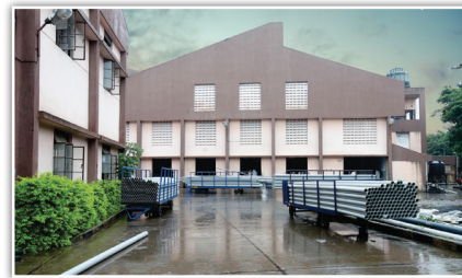
Dadra - Silvassa (Pipes & Water Tanks)
