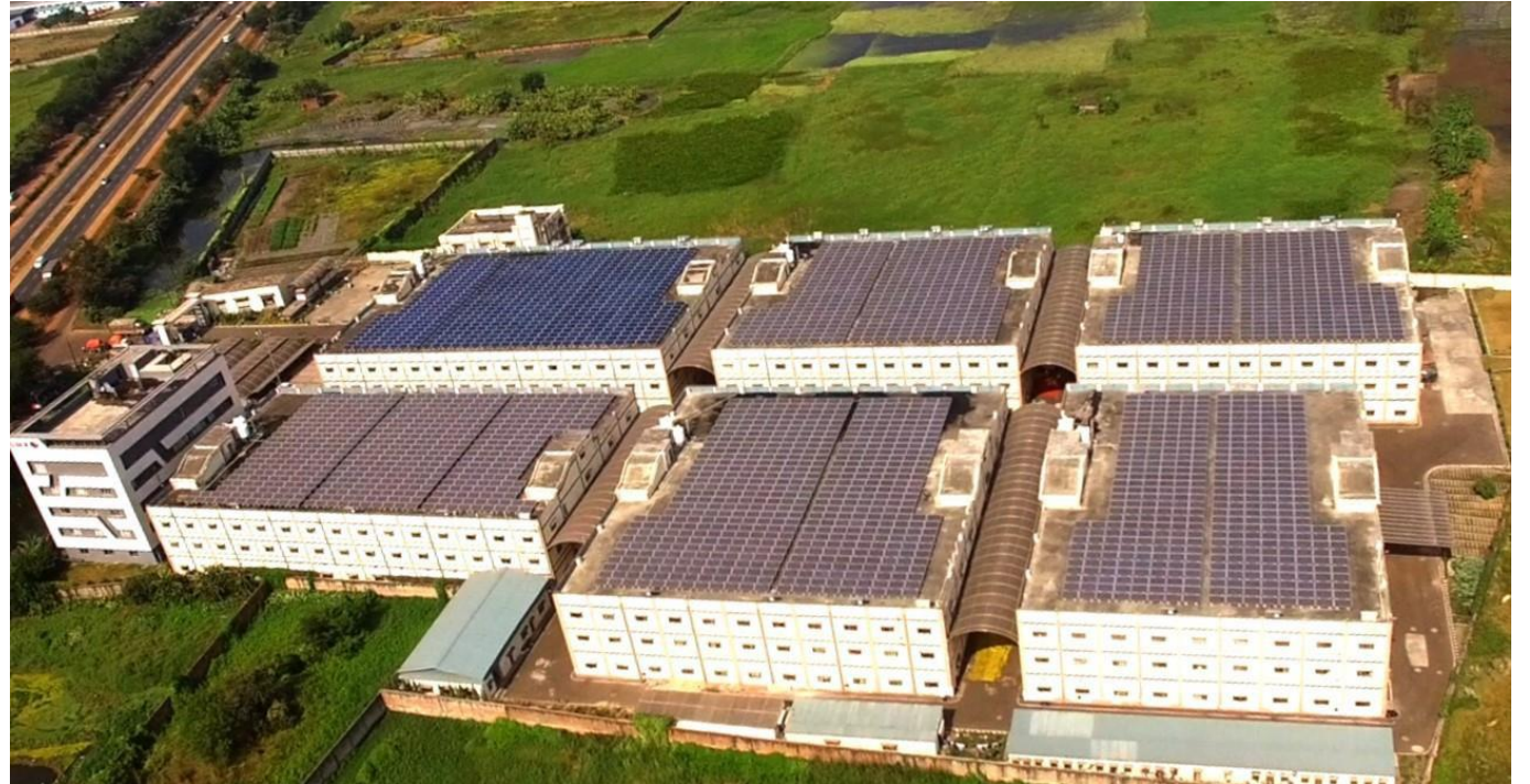
Rooftop solar power plant at Dankuni unit
