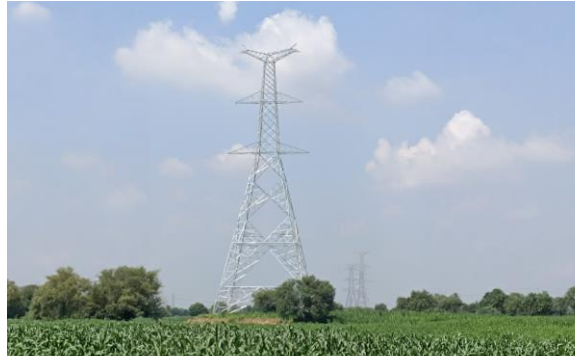
Koppal-II PS – Narendra 765 kV D/C line, Karnataka
