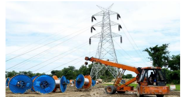
400 kV Quad New Butwal to Indian Border Transmission Line Project, Nepal
