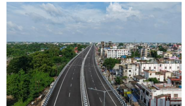
Begusarai elevated road project, Bihar
