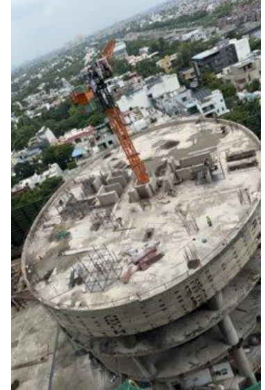
Column re-barring work in progress
