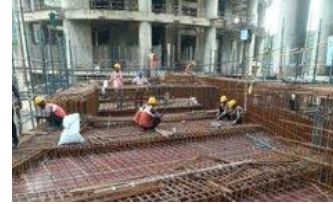
Slab shuttering work in progress
