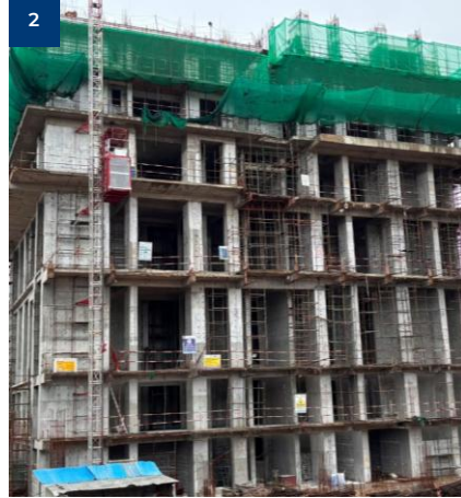
4th floor slab of Tower 3 & 5 completed. 5th floor slab in progress
