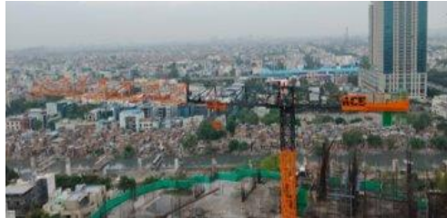
Installation of tower crane in progress
