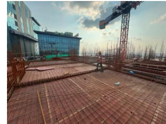
Slab reinforcement and shuttering work in progress
