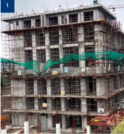
1st floor slab of Tower 1 & 2 completed. 2nd Floor slab in progress
