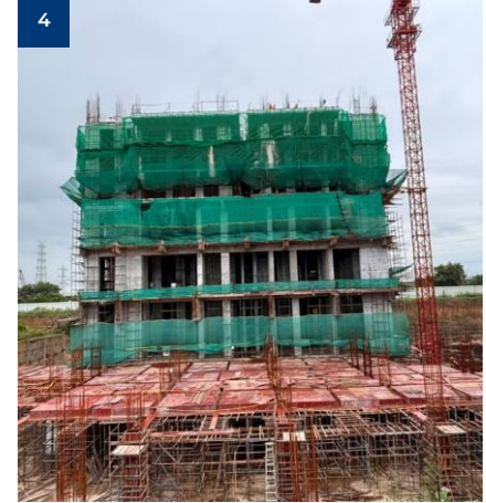
4th floor slab of Tower 6 complete. 5th floor slab in progress
