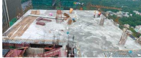
Terrace level slab casting in progress
