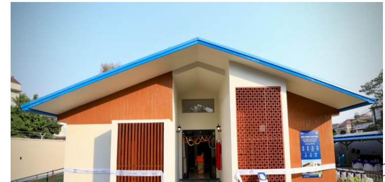
Pioneering sustainable future with Zero Energy Building Solutions (Nest-In)
