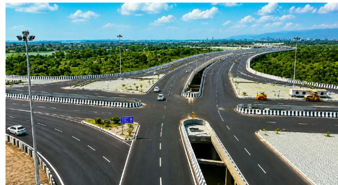
Stilt Bridge SBR-9, Eastern Connectivity - Maharashtra
