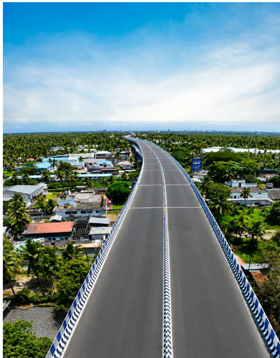
Aroor-Thuravoor 6-Lane Elevated Corridor (12.752 kms.) - Kerala
