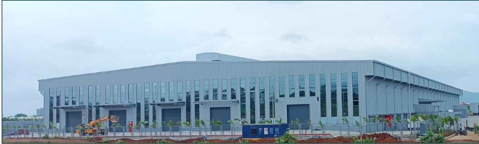
North-West View of the Plant
