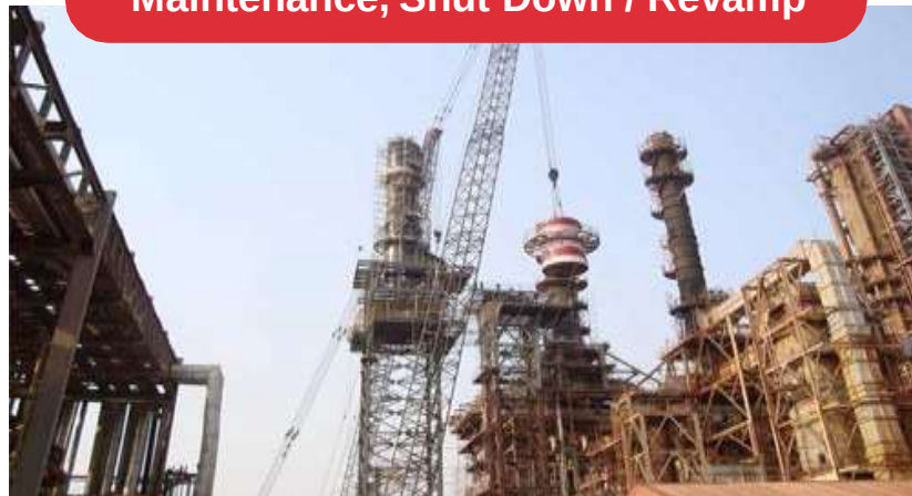
Maintenance, Shut Down / Revamp
