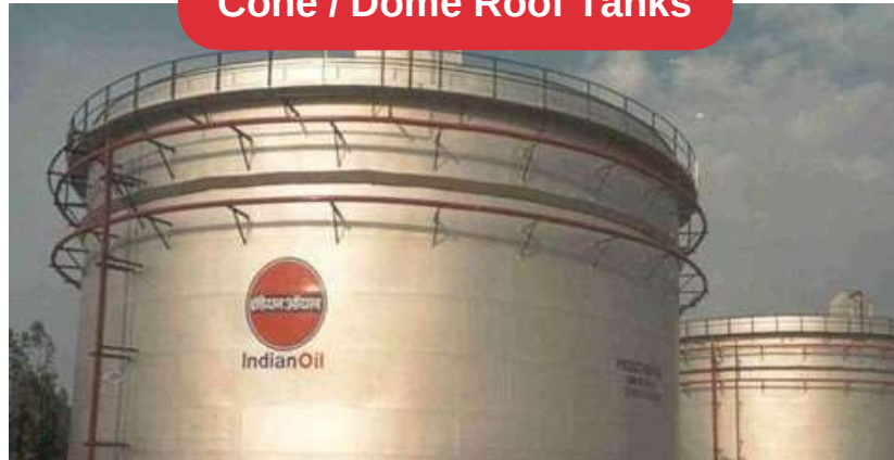
Cone / Dome Roof Tanks
