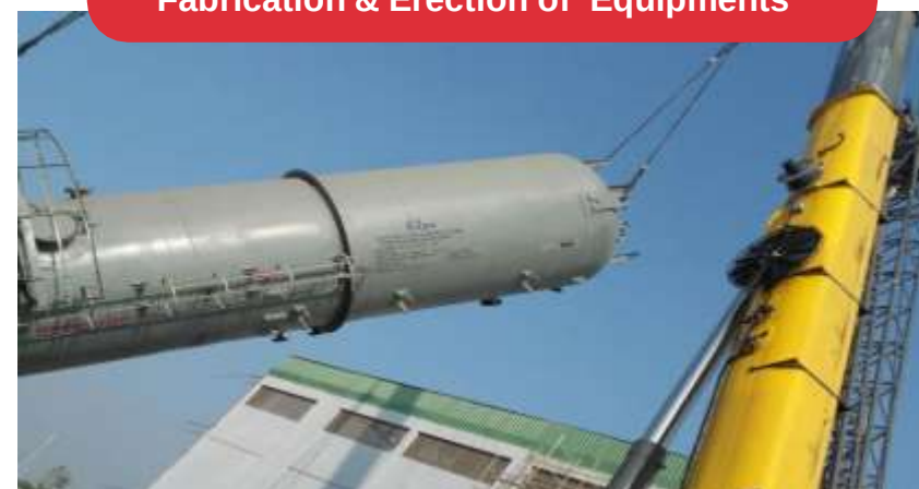
Fabrication & Erection of Equipments
