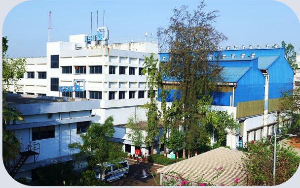
Dedicated spares manufacturing plant
