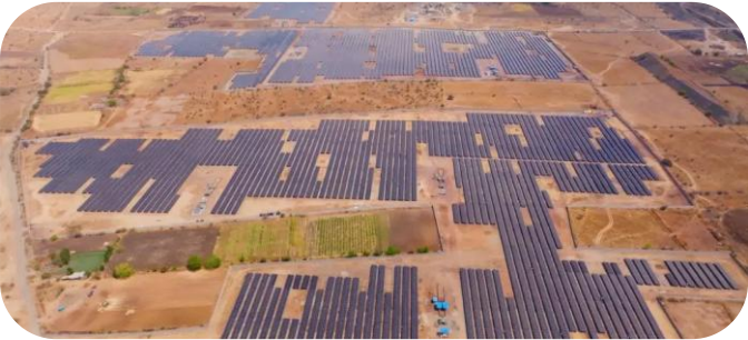
Open access 150MWp project (Sunsure)
