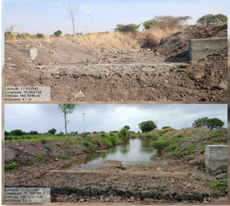
Soil & Water Conservation - Deepening and widening of water stream
