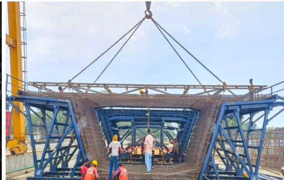
AYODHYA BYPASS 4200 meter bridge over Saryu River UP's Longest
