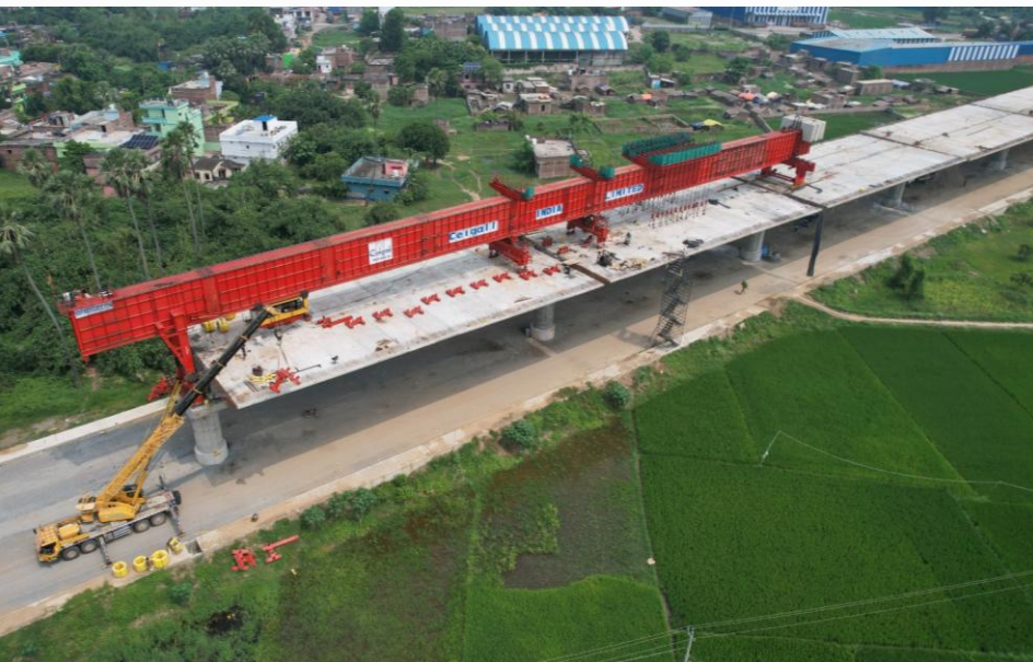
DANAPUR BAHITA PROJECT I India's longest four-lane elevated corridor, spanning 19.87 kilometers
