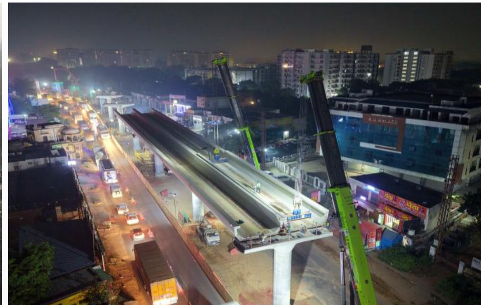
AGRA METRO Design and construction of 3 Agra stations
