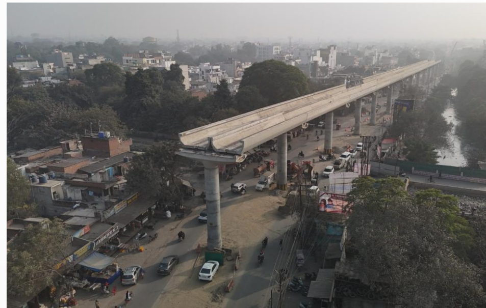
KANPUR METRO construction of 5 elevated stations
