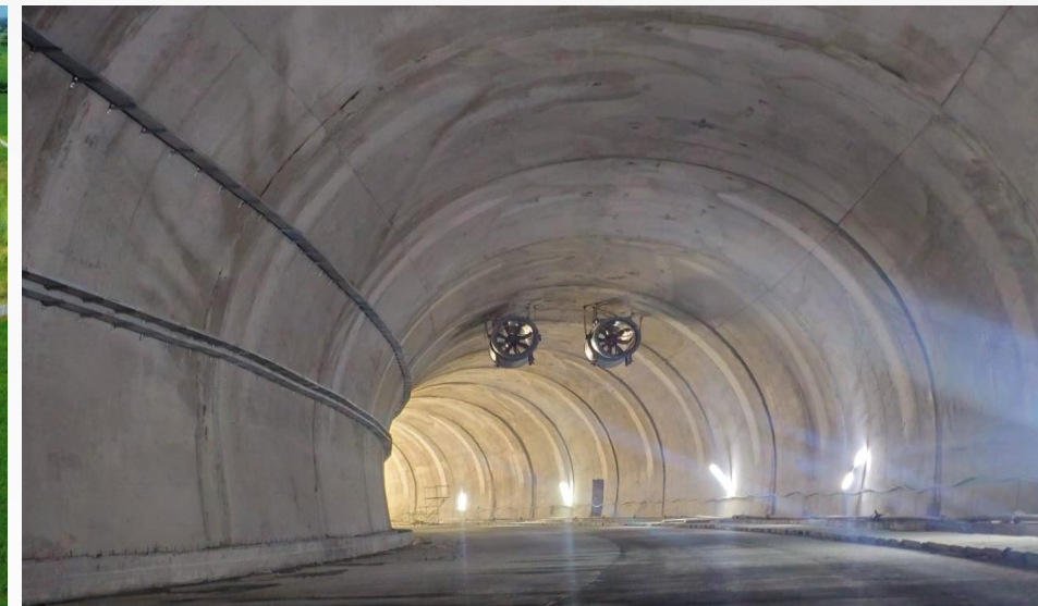
RAMBAN-BANIHAL PKG II twin tube tunnel of 6 Km in J&K
