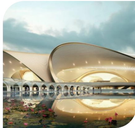
Navi Mumbai International Airport
