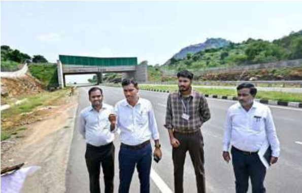
R. Murugaprakash, Project Director, NHAI, reviewing construction work on Madurai Ring Road connecting Vadipatti-Thamaraipatti in Madurai on Tuesday. G. MOORTHY
