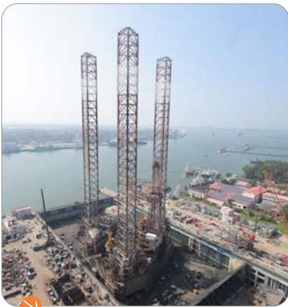
Oil Rig Upgrades, Repair Projects, and Conversions
