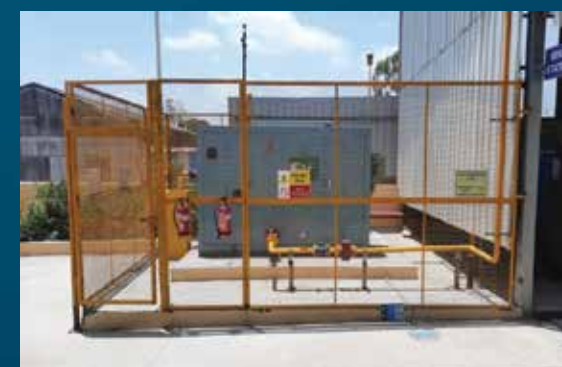
Air Pollution -MNGL Station
