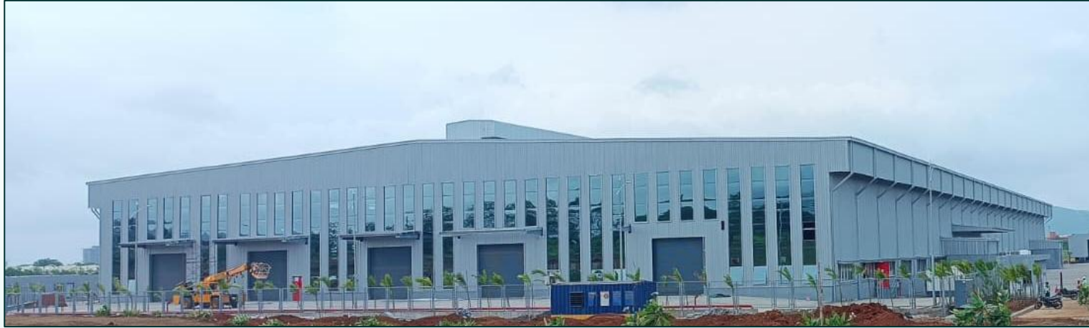
North-West View of the Plant
