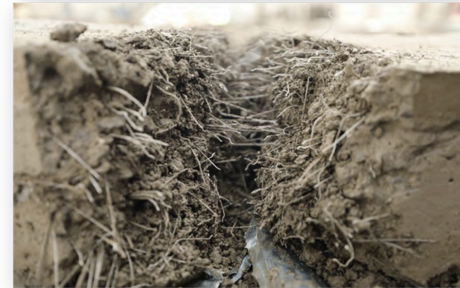
Steel Fiber Reinforced Concrete Flooring
