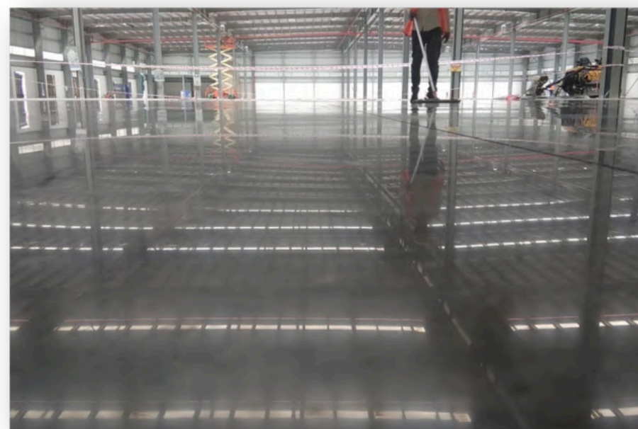
Concrete Polishing and Densification
