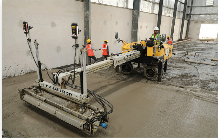
FM1/ FM2 Grade - Laser Screed Floors
