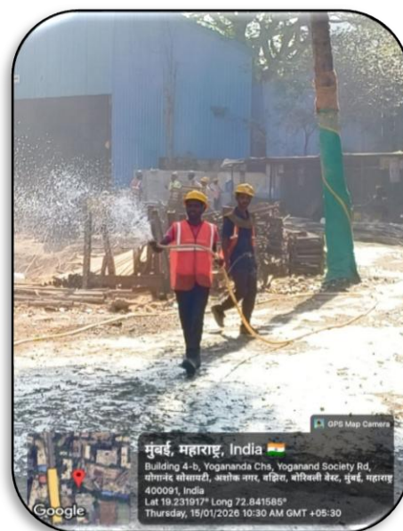
Water spraying for dust suppression
