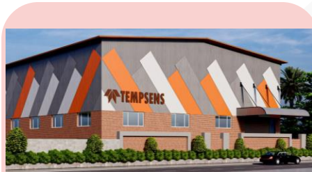
New plant within existing Unit 6
