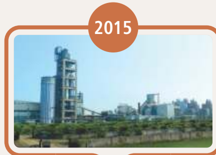
Integrated Unit at Durg
