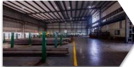
Covered Raw Material Yard
