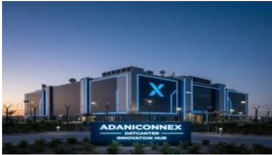
Adani Connex Data Center
