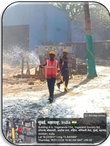
Water spraying for dust suppression
