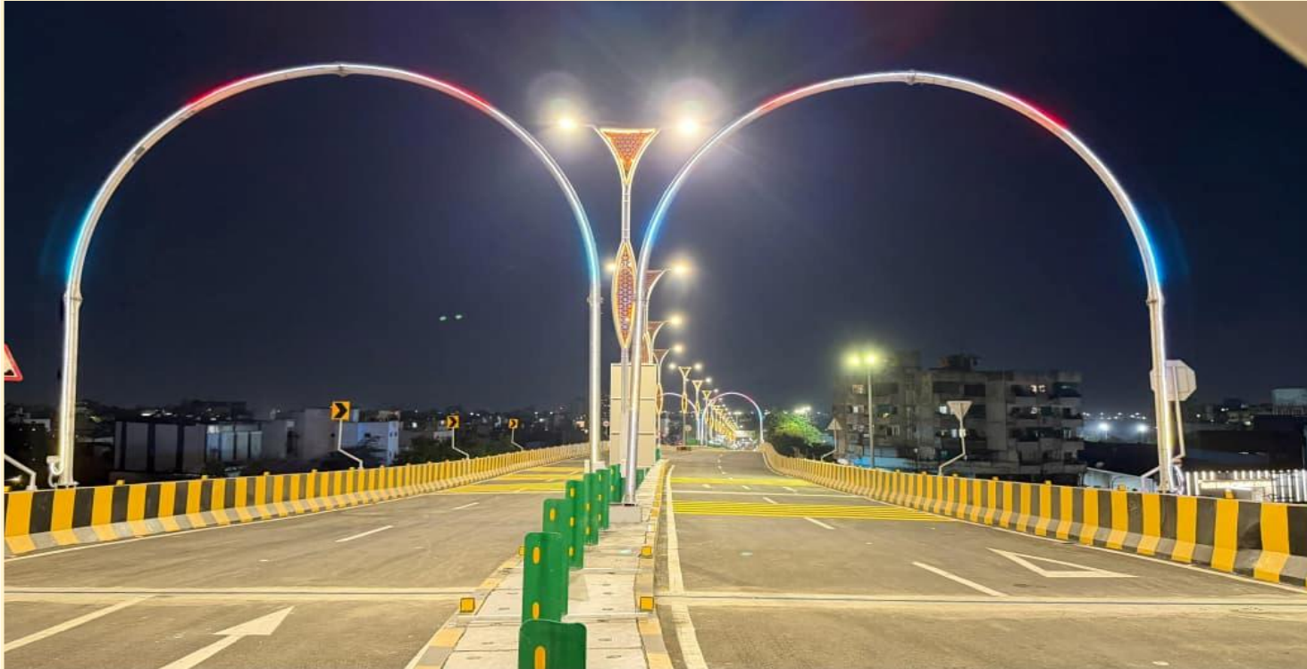
Dipti Signal Road Over Bridge in Nagpur
