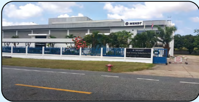
Wendt Grinding Technologies Ltd, Thailand
