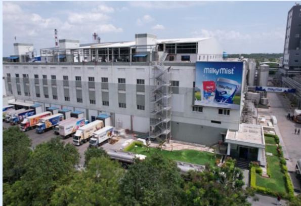
PERUNDURAI, ERODE FACILITY
