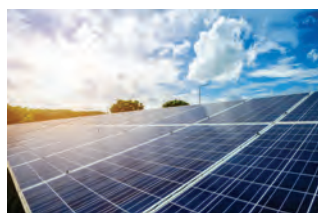
Copper in Solar plants
