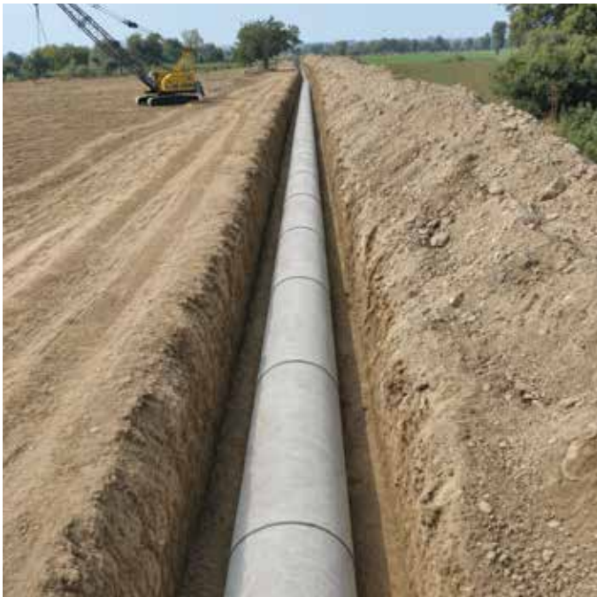
1700 mm dia PCCP pipeline laying for Pressurised Piped Distribution Network of Varkhede Londhe Irrigation Project, Jalgaon, Maharashtra
