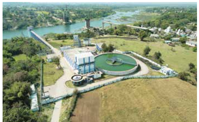
Intake well & 31 MLD Water Treatment Plant in Behdaghat project in Jabalpur District in Madhya Pradesh
