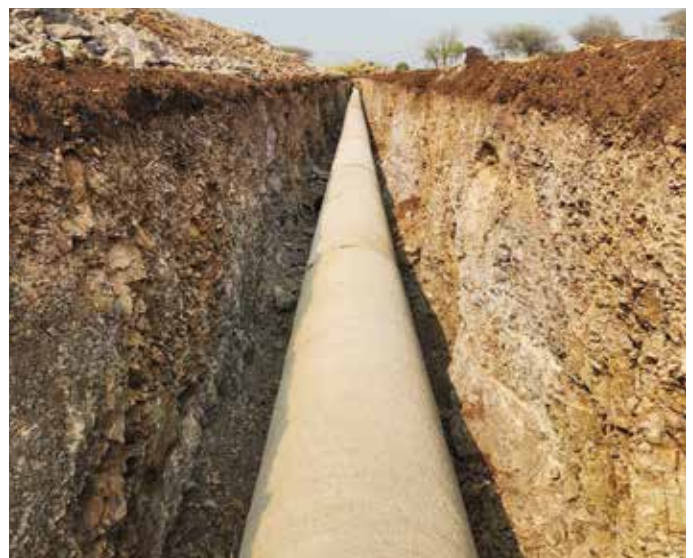
800 mm dia PCCP pipeline laying for Piped Distribution Network of Dahigaon Lift Irrigation Scheme, Solapur, Maharashtra.
