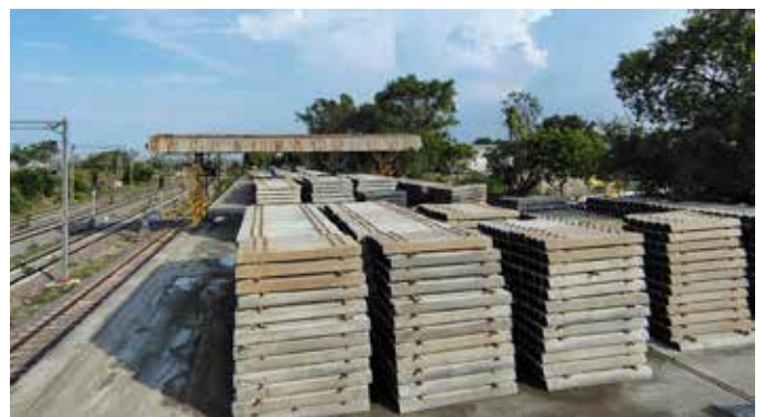
Wider Base Sleepers Confirming to RDSO Drawing No. RT-8746 Stacked on Siding Yard for Loading into Wagons/Trucks at Karari-II, in Uttar Pradesh
