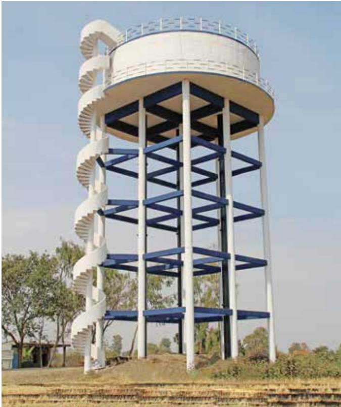
3.6 lakhs Ltr. capacity Break Pressure Tank (BPT) at Buldhana Water Supply Scheme, in Maharashtra
