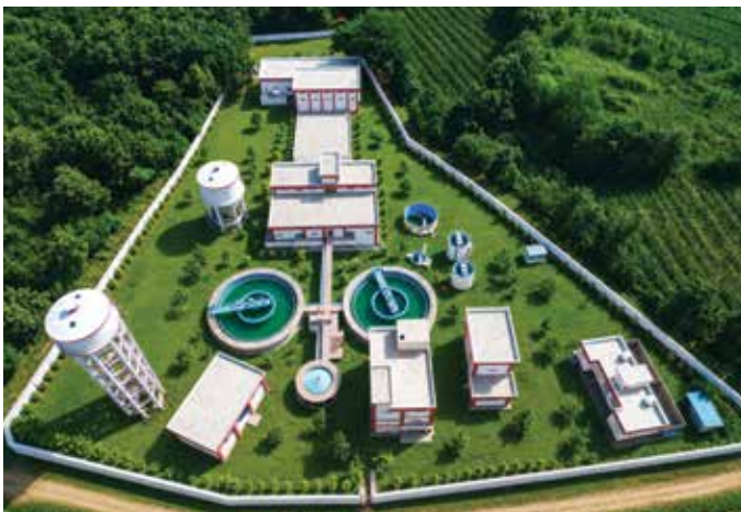
9.2 MLD Water Treatment Plant for Gajapati Water Supply Scheme, Odisha
