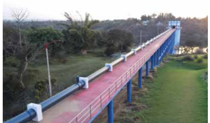
Intake well with approach bridge of 3 mtr wide and 160 mtr length for Raw water pumping main in Bhedaghat 5B project in Jabalpur District in Madhya Pradesh.
