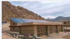
5kW Roof and Mud Walls In Ladakh being tested for superior thermal insulation
