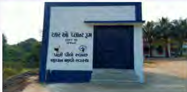
RO Room and RO with Chilling unit at village Charetha, Taluka Mangrol, District Surat
