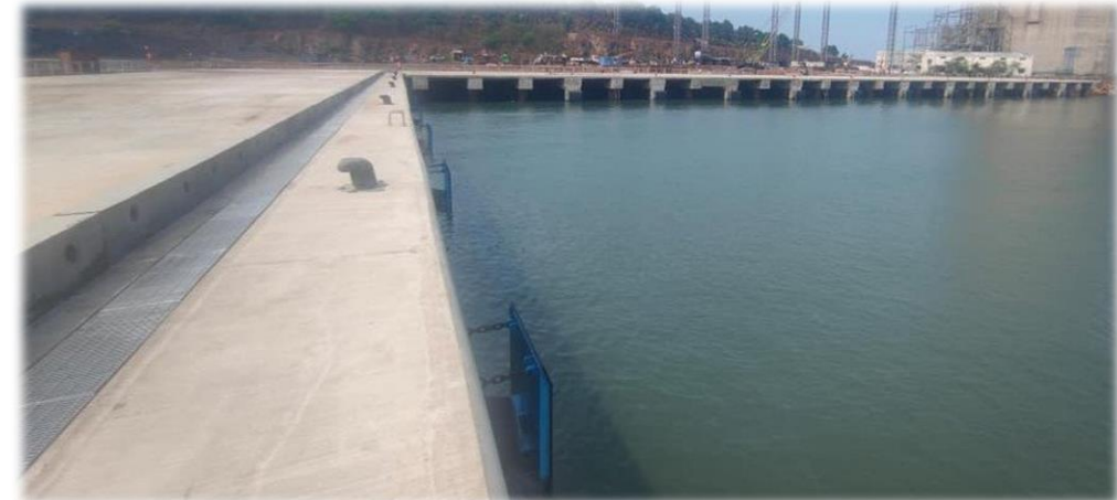
Expansion work at Jaigarh Port
