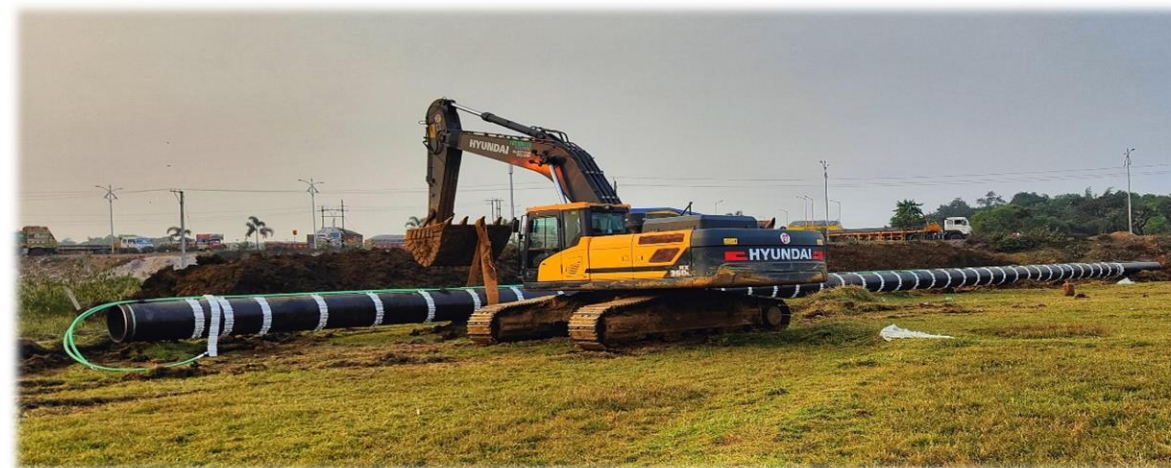
Setting up slurry pipeline
