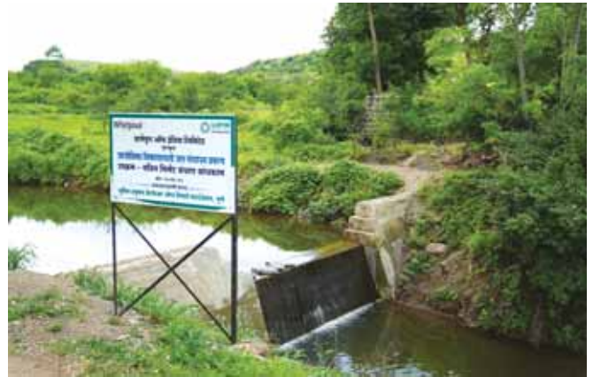
Construction of cement nala bund at Kendur village, Pune
