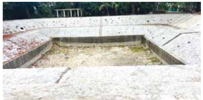
Completion of pond rejuvenation at Thirubuvanai kuttai, Puducherry
