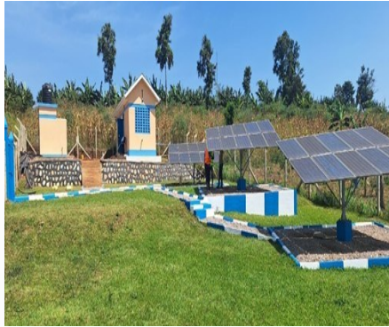
Drinking Water Supply Project in Uganda
