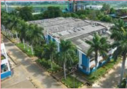
Plant 1, Bonthapally 79 Kms from Hyderabad Airport, Telangana
