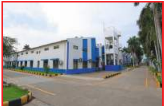
Plant 4, Bonthapally 79 Kms from Hyderabad Airport, Telangana
