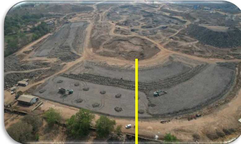
Geomembrane Faced Rockfill Dam
