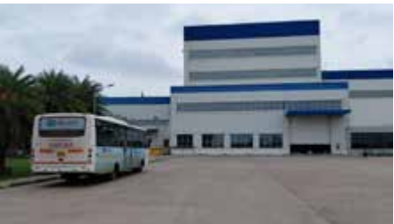
Ankhi Unit-V, Gujarat Capacity (MVA) : 15,780
