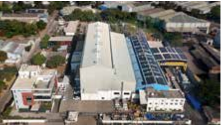
Anand Unit-I, Gujarat Capacity (MVA) : 9,360
