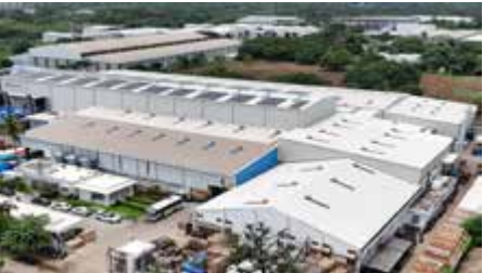
Anand Unit-II, Gujarat Capacity (MVA) : 6,660
