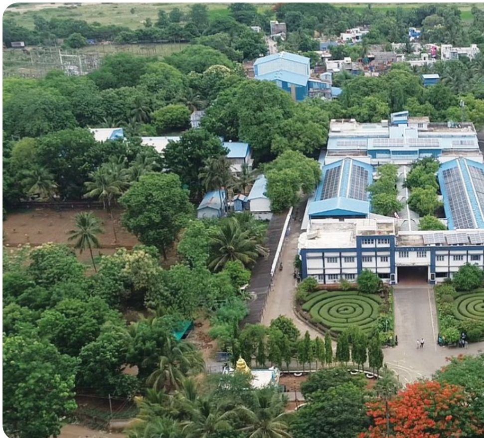
→ Puducherry plant integrated rooftop solar installations.
