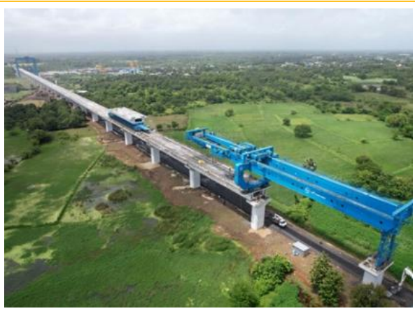
Mumbai Ahmedabad Bullet Train [Chemicals & Aggregate Supply]
