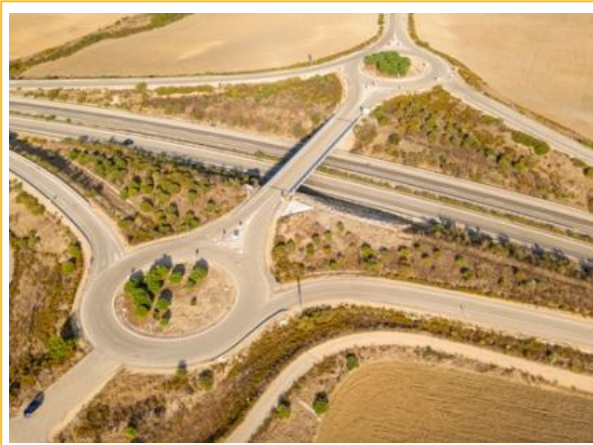
Chennai Peripheral Ring Road [Aggregate supply]
