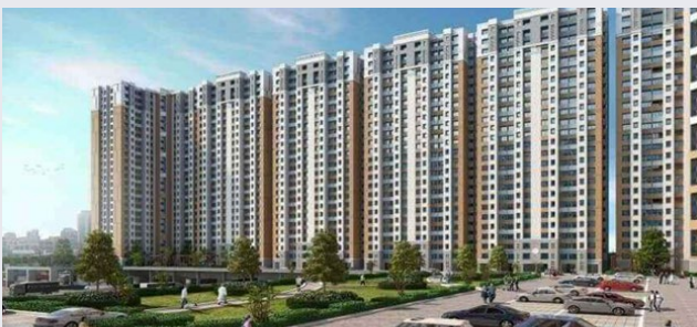
[Aggregates, chemicals, walling, flooring, plumbing supplies to a large PMAY project in Navi Mumbai]
