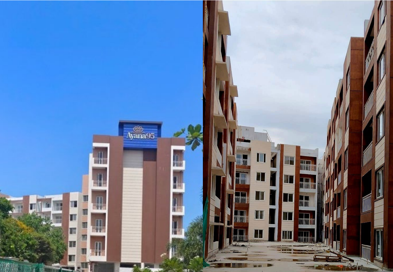
DaaS delivered project in Chennai
