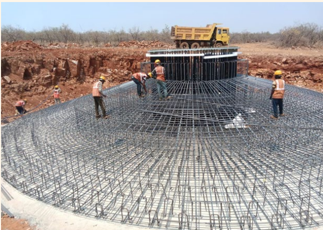
[Cut & bend steel supplies to a premier wind energy client]
