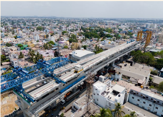
[RMC supply to a listed EPC contractor for Chennai Metro]
