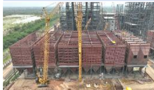
Junction Tower Structure erection
