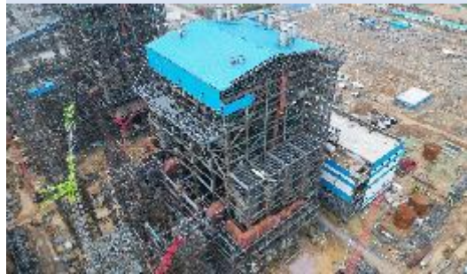
Front View of MPH & Boiler
