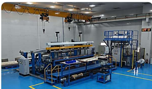
Bushing Winding hall
