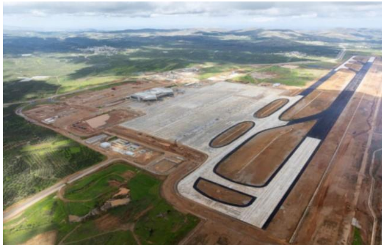
Airside Pavement Works
