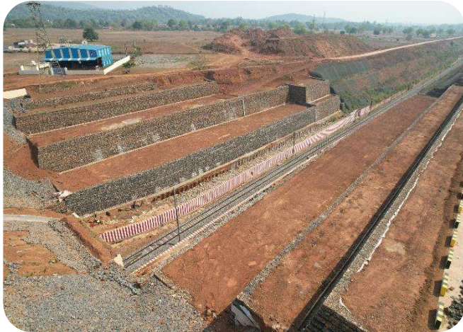
Slope Retaining Works
