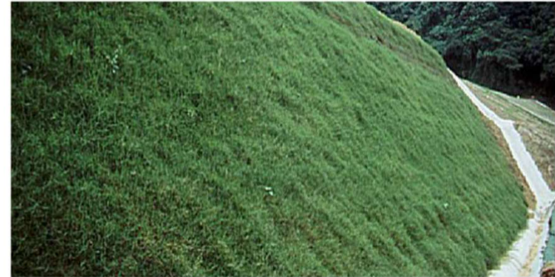
Slope Protection works for a project
