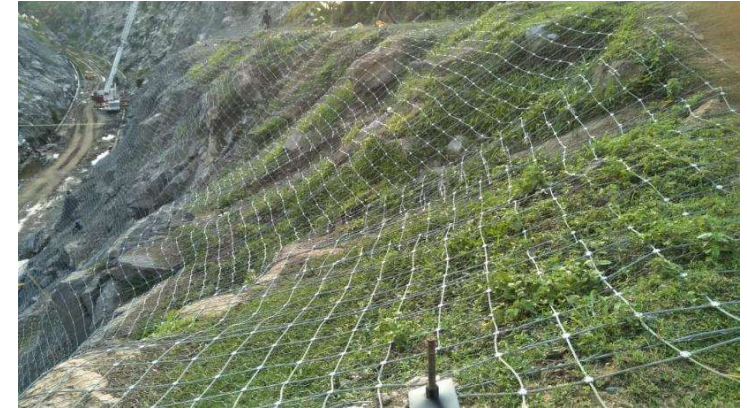
Rockfall Protection works for a project in state of Jharkhand
