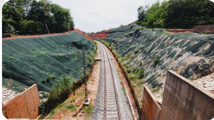
Slope Protection works
