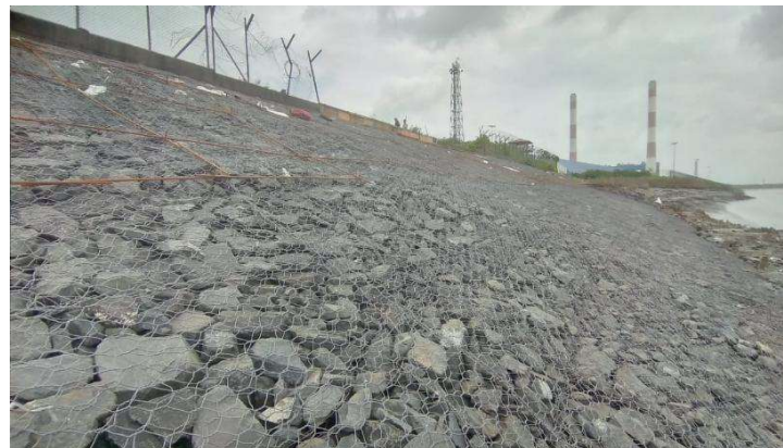
Coastal Protection works for a project in State of Gujarat
