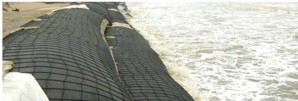
Coastal Protection works for a project
