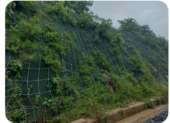
Slope Protection Works
