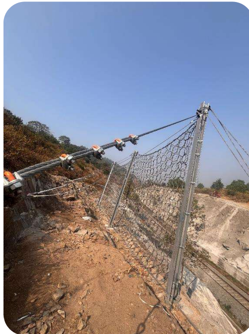
Rock Fall Barrier Works
