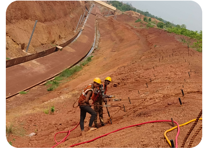
Slope Protection works
