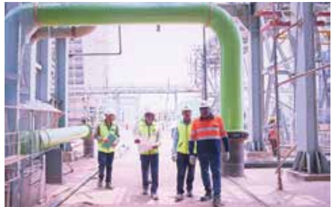
▲ Mr. Arun Vijay, President – Projects, reviewing the progress at the Gopalpur Project site.
