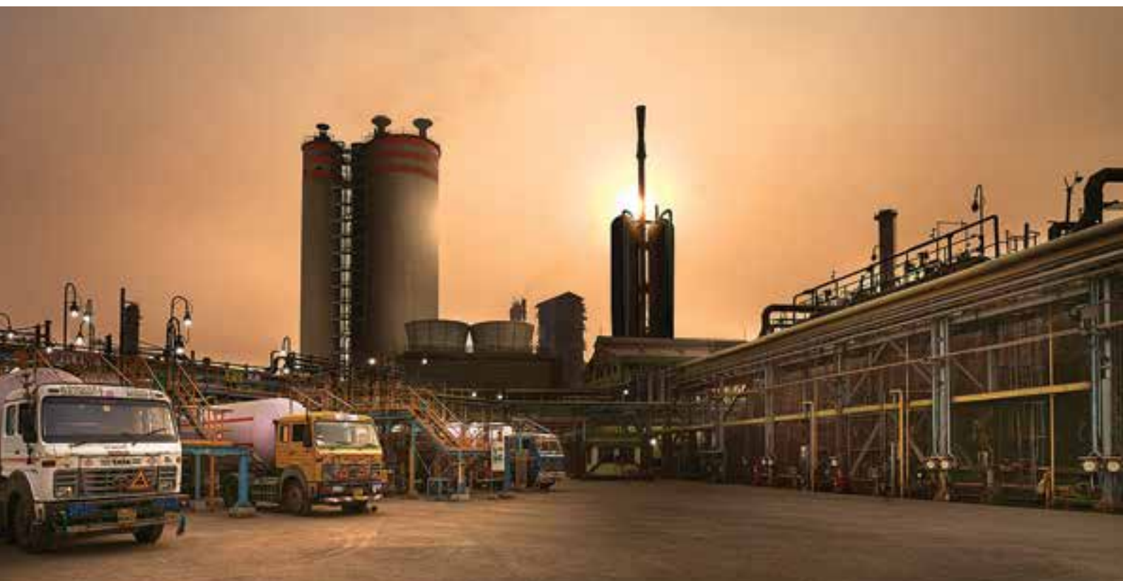
▲ Sunset view of the K-1 plant taken from Propylene unloading area, with Prilling Tower and Nitric Acid plants seen in the background.
