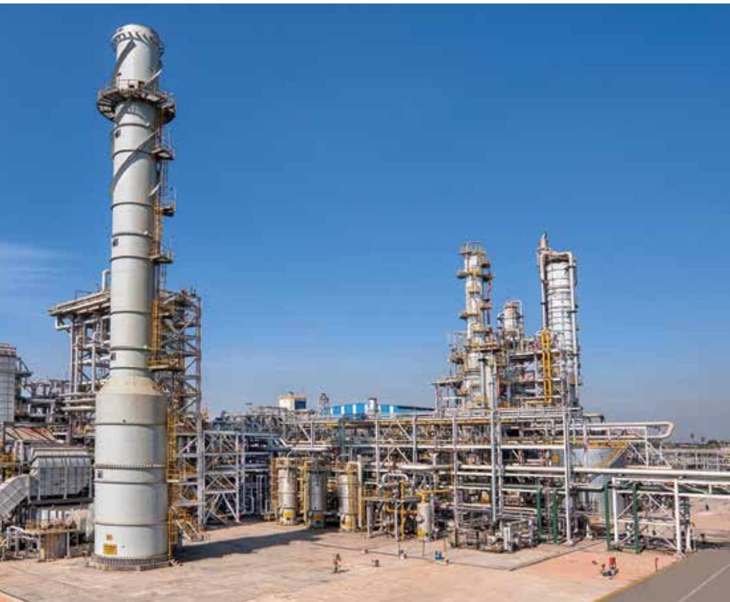
▲ State-of-the-art 1,500 MTPD Ammonia plant powered by KBR KRES technology, aligned with the nation's Aatmanirbhar Bharat mission.
