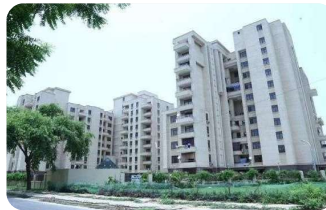
Residential accommodation for NHA staff at Sector17, Dwarka, New Delhi
