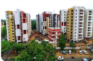
Construction of 222 Flats at Keelandev Tower, Bhopal for MP Housing & Infrastructure Development Board
