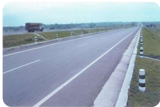
Maintenance of NH-19, (earlier NH-2) Barwa Adda –Panagarh Section (KM 398.75 –KM 512.00) in the state of Jharkhand & WestBengal
