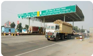
Development & Operation of Bikaner- Suratgarh Section of NH-62 (earlier NH-15) in the state of Rajasthan
