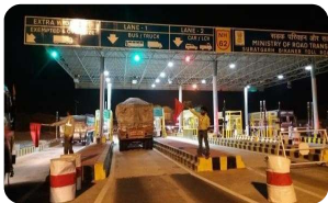
Development & Operation of Bikaner- Suratgarh Section of NH-62 (earlier NH-15) in the state of Rajasthan
