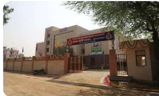
Construction of Police station & Residential Quarters, Hari Nagar, Delhi for MHA, Delhi Police through RITES Ltd.
