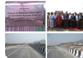
Construction of 2 lane flyover on Guwahati Bypass of NH-115 (earlier NH-37) in the state of Assam
