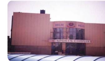
Police Station & Residential Quarters at Kondli, New Delhi for MHA, Delhi Police through RITES Ltd.
