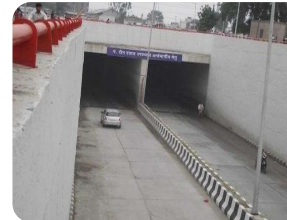
Construction of RUB at Badli, New Delhi
