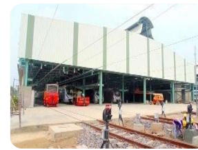
Construction of Metro Rail Depot, Kalindi Kunj, New Delhi
