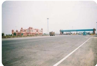
Toll Plaza construction at Delhi –Agra, NH-44 (earlier NH-2)
