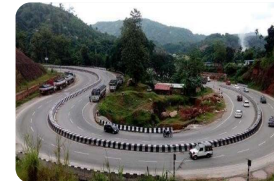
Widening & Strengthening of existing National Highway from 2 lane to 4 lane of Sonapur to Guwahati section of NH-115 (earlier NH 37)
