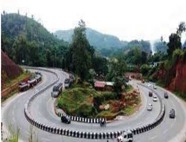
ROADS & HIGHWAYS – CONSTRUCTION/EPC
