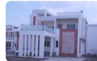
Construction of Director/Dean Bungalow, QIP Centre & accommodation for SPA at Bhopal
