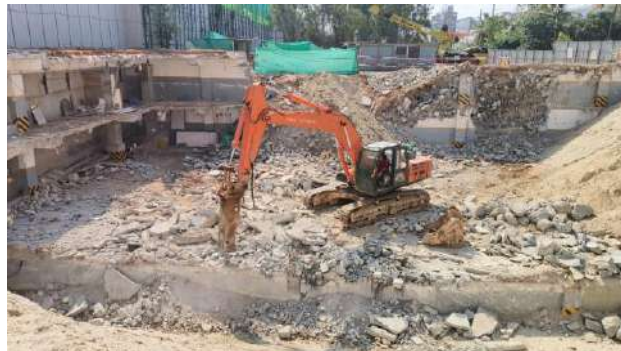
Commencement of construction
