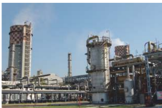
VIJAIPUR I & II PLANT
