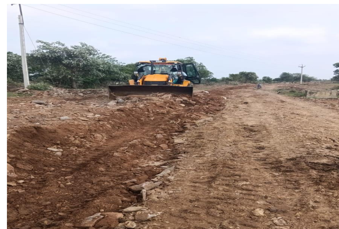
Road development work at Nimbahera
