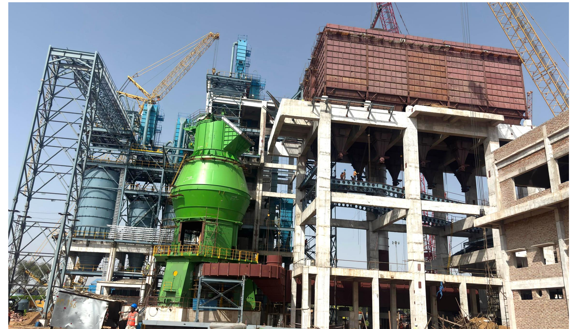
Cement Mill & Building
